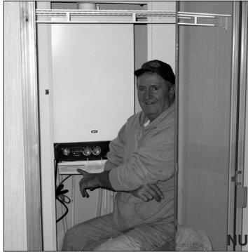
**The Baxi Luna wall-hung boiler is so compact it can fit in the back of a bedroom closet.**
